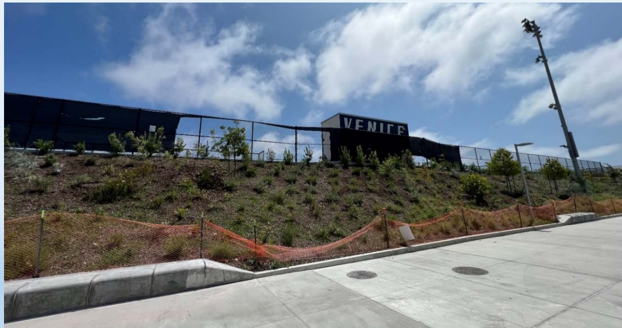
Venice HS – Football Field Bleacher Berm - (OIG Photo– August 11, 2023)
